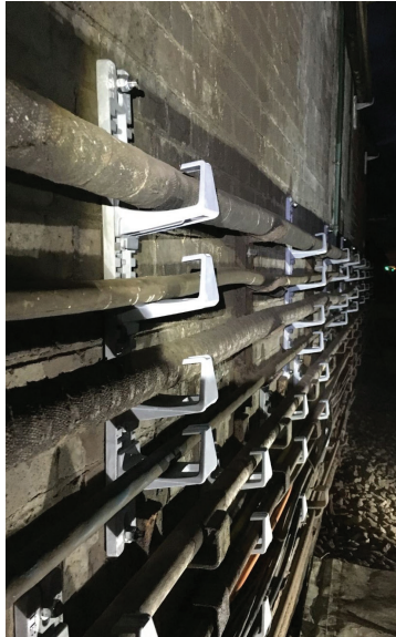
INSTALLATION ON LONDON UNDERGROUND
