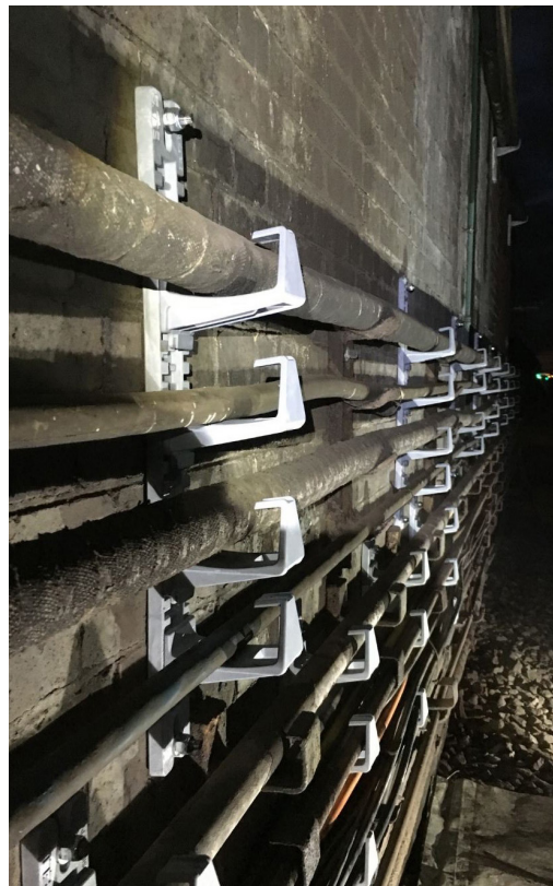
INSTALLATION ON LONDON UNDERGROUND
