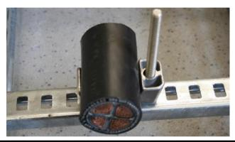
3) Locate the other half of the cable clamp. Secure with a nut and washer (not supplied) to the support structure and tighten.
