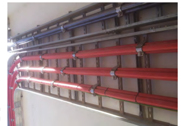
THE LATERAL LOAD RATING OF A CLEAT CAN BE USED TO SPECIFY CLEATS BASED ON CONTINUOUS LOADING, SUCH AS MOUNTING CLEATS ON A SIDE.
